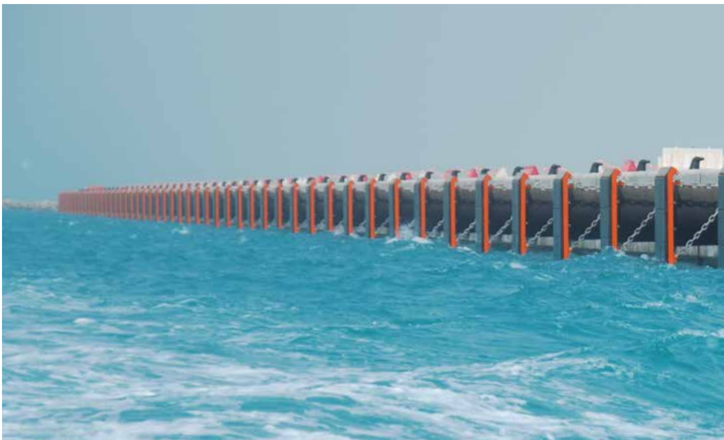
Container Terminal, Khalifa Port, Abu Dhabi
