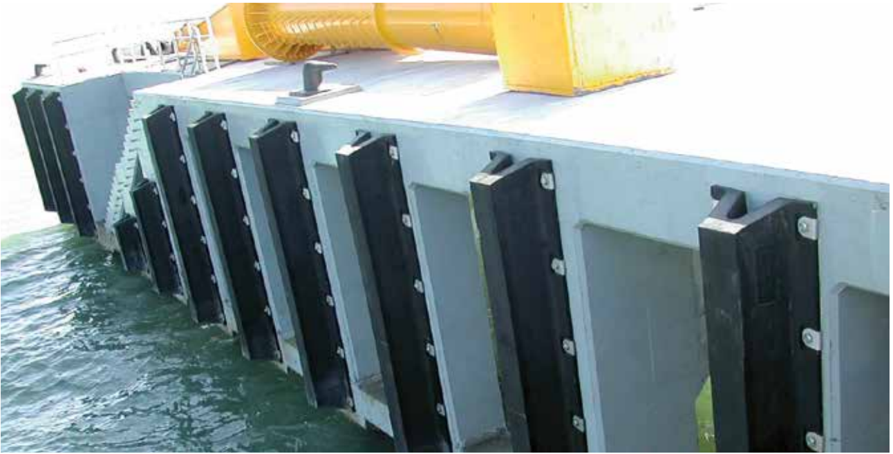
Small Craft Jetty, Port Klang, Malaysia
